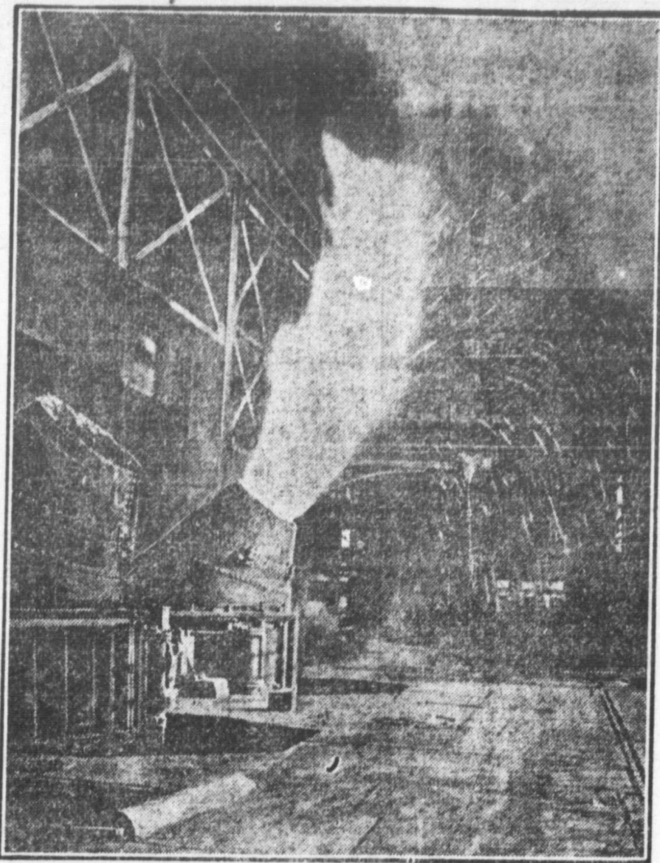
A Bessemer Furnace at Work Preparing Steel.
